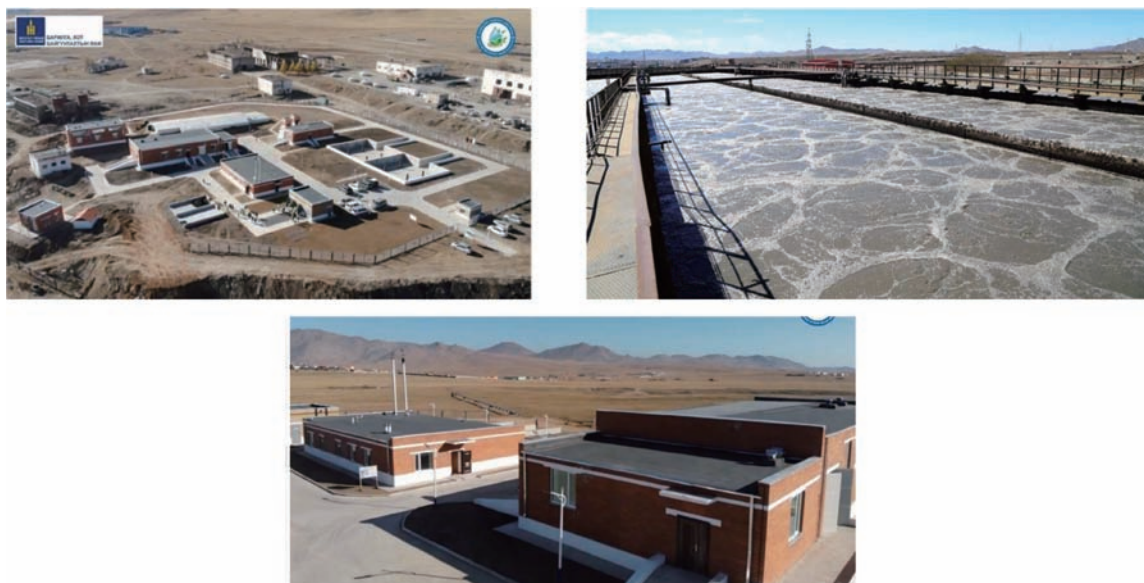
Figure 14. The new water supply and sanitation infrastructure for residents of Dalanzadgad Soum
